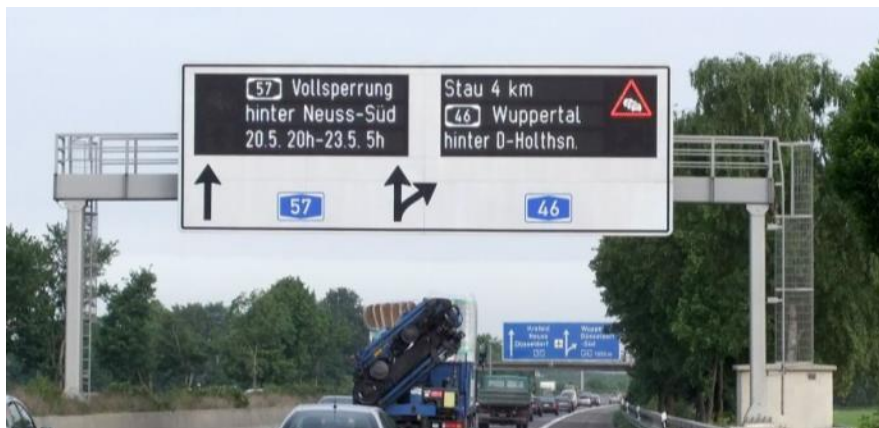
Figure 1 – dWiSta: dynamic sign post with integrated traffic information [THOMAS Verkehrstechnik]
